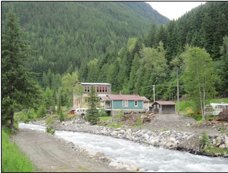
Photo 1. View of the historical town of Sandon, with Carpenter Creek in the foreground.
