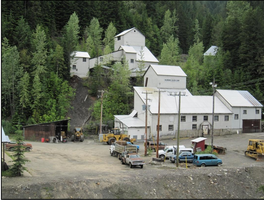
Photo 6: View of the Klondike Silver mill site at Sandon; the coarse ore chute is shown in the center background, the assay lab in the top right; the office facilities are located to immediate left of photo.dsa
