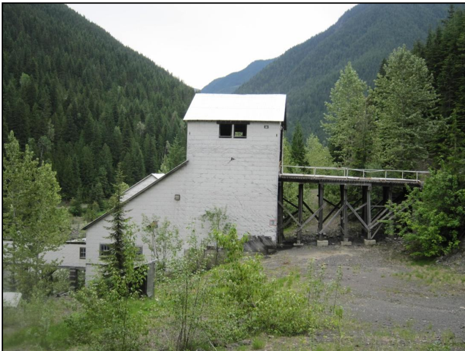
Photo 7: View looking up the Carpenter Creek valley with the coarse ore bin shown in the foreground.
